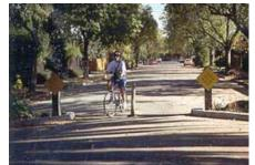
Another method commonly used to create road closures is installing curb extensions to the roadway.
