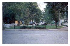
Road closures are very effective at lowering traffic volumes on the roadway. Cut through traffic can be greatly reduced through the use of full closure. It is common to use full closures to limit the amount of traffic on a residential street that was connected to a main street. By closing the connection to the main street, the traffic that previously used the residential street to connect to the main street would diminish thereby decreasing the overall
