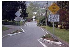
attention to be paid to the area which allows for safer pedestrian travel. Some designs may allow drivers to cut across and take a straight path through the angle point. This design is advantageous for emergency vehicles as they do not generally need to slow down for these zones.
