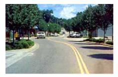
Chicanes are offset curb extensions that form S-shaped curves which cause a deviation in the vehicle's path of travel. They realign the road horizontally to force the driver to alter their path causing them to slow down. Chicanes can also be created by alternating parking between each side of the road. Chicanes can be effective at reducing vehicle speeds without the noise and inconvenience of speed bumps or other methods.
